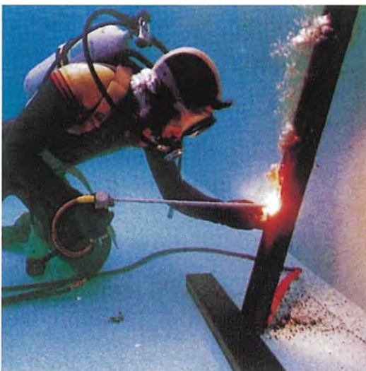
Under water cutting 水中切断
