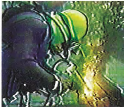
Under water cutting 水中切断
